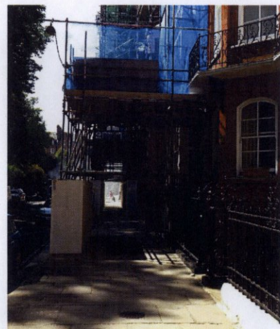
Proposed scaffolding & gantry as per photograph.
